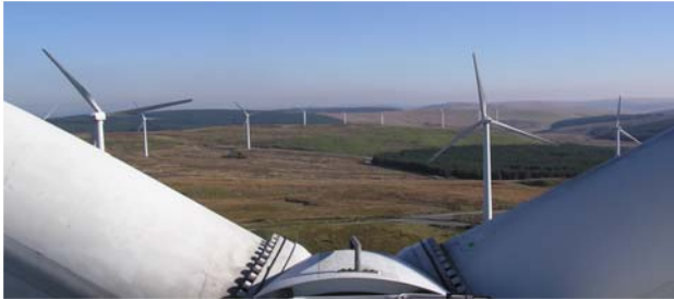
Figure 1: A Typical Wind Farm
